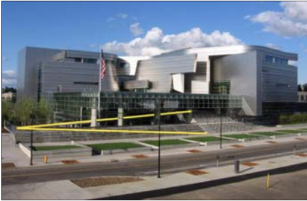
Plinths often require complex access routes
